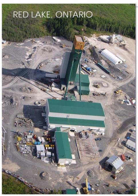
Goldcorp's Mine **Expansion & Shaft Project included** the construction of the 6,314' McEwen Shaft, retrofit and upgrade of the existing mill to 1,200 tpd, a new shop and office facility, water treatment plant and material handling interface for increasing mill throughput.
