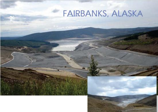
Kinross Gold's Fort Knox Mine near Fairbanks is an open pit with carbon-incolumn, heap leach and gravity processing.
