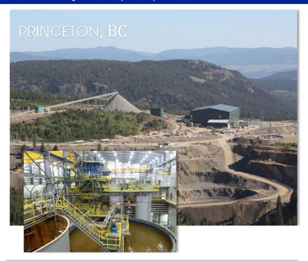
Copper Mountain Mining Corporation's 35,000 tpd mine is a conventional open pit operation with crushing, grinding, flotation, and concentrate handling processing. Merit provided Project and Construction Management services that included a concentrator building, truck shop, 138kV power line and substation.
