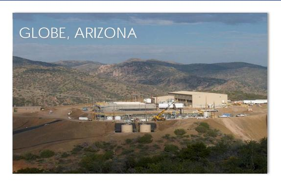
Carlota Copper Corporation's (Quadra Mining Ltd.) mine is an open pit 24,000 tpd run-of-mine heap leach with solvent extraction / electrowinning plant, heap leach pad and ponds and truck shop.
