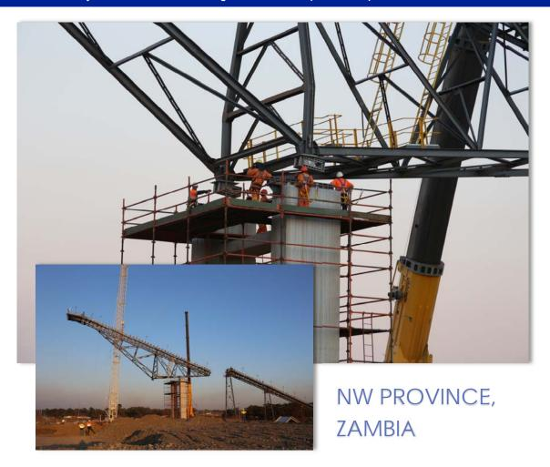
Merit provided Construction Management services for the recovery work on Conveyor 3 following a structural failure. Merit services included site coordination of the contractors, quality control and assurance, oversight of material, expediting, and contractor-engineer-vendor scheduling.
