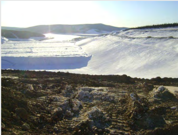
Heap Leach - Stage 3 Construction - 2011
