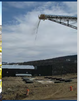
First Ore to Primary Crusher and Stockpile
