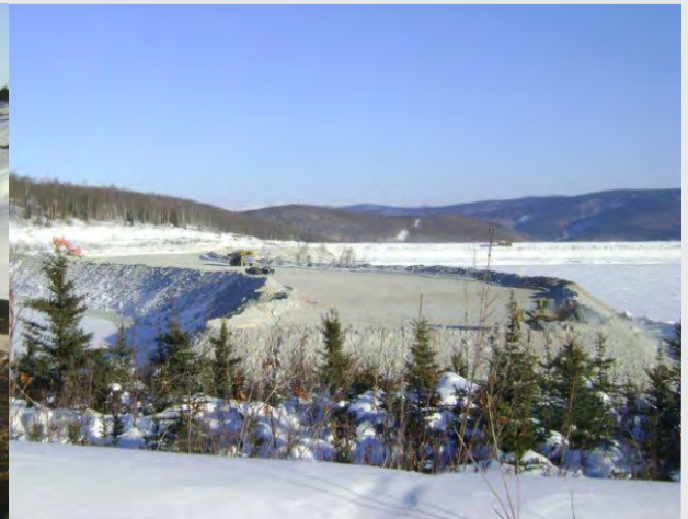
Tailings Storage Facility - Jetty Construction - 2011
