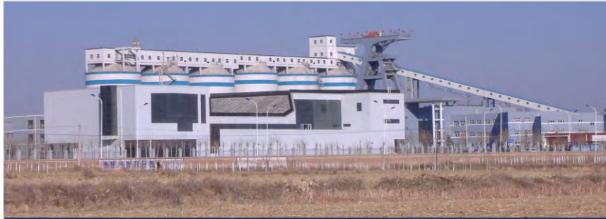
Employee Training Building No#1 Service Hoist Raw Coal Silos
