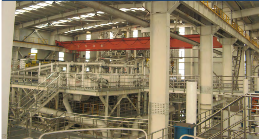
Inside Coal Wash Plant
