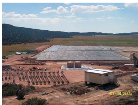
Leach Pad Liner
