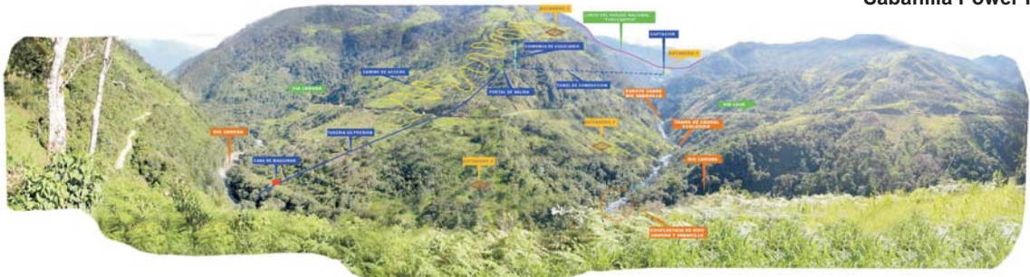
Sabanilla Power Project
