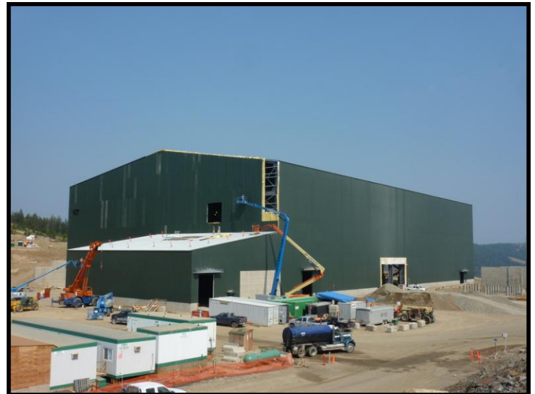
Concentrator Building Outside Cladding Now Complete
