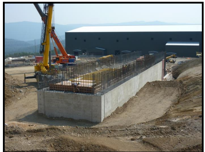
Concentrator Building Rear View with Reclaim Tunnel
