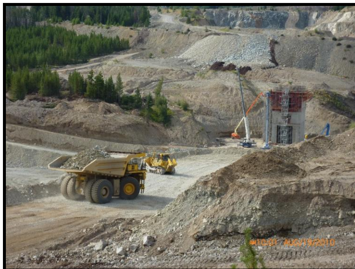
Komatsu 830E hauling fill material to crusher area
