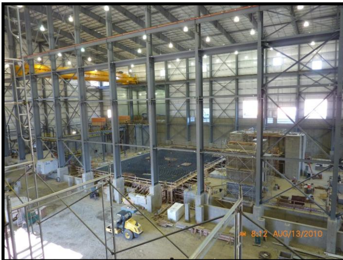
Concentrator Building Interior View
