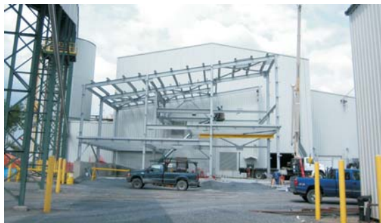
Steel Erection - New Shop/Office Facility
