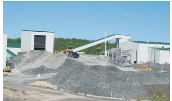
Approach Ramp - New Truck Dump Facility
